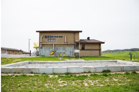
Odor Control System
