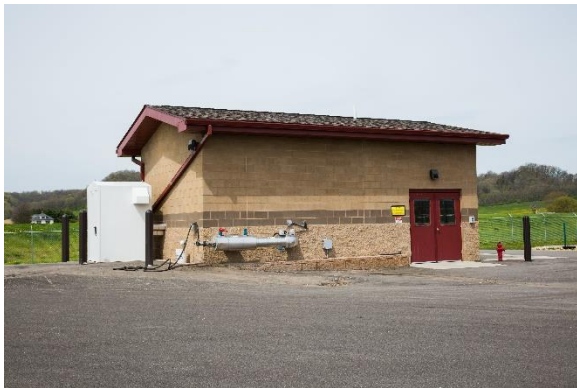
Hauled Waste Receiving Building
