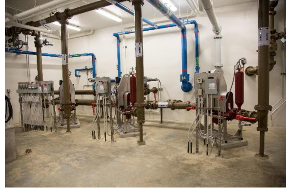
Primary Sludge Pumping
