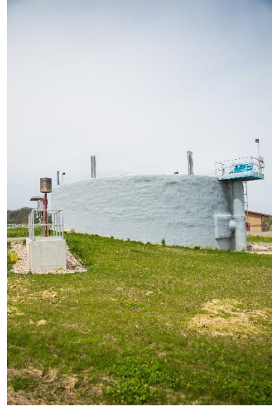
Anaerobic Digester and Flare
