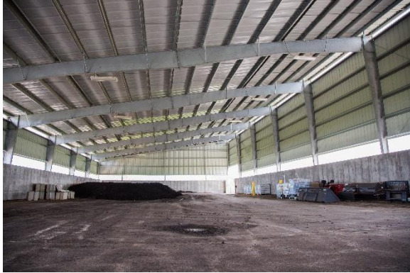
Biosolids Cake Storage Building
