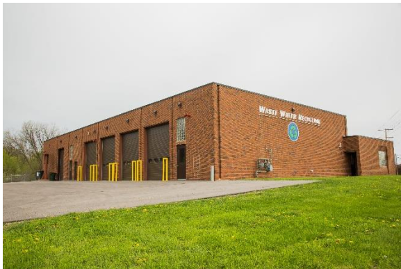
Existing Administration Building
